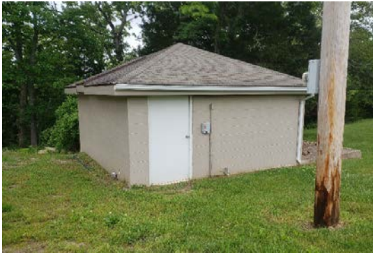
Well No. 1 Well House
