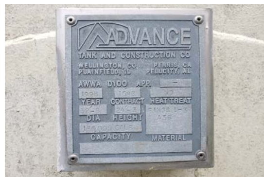
Water Storage Tank
